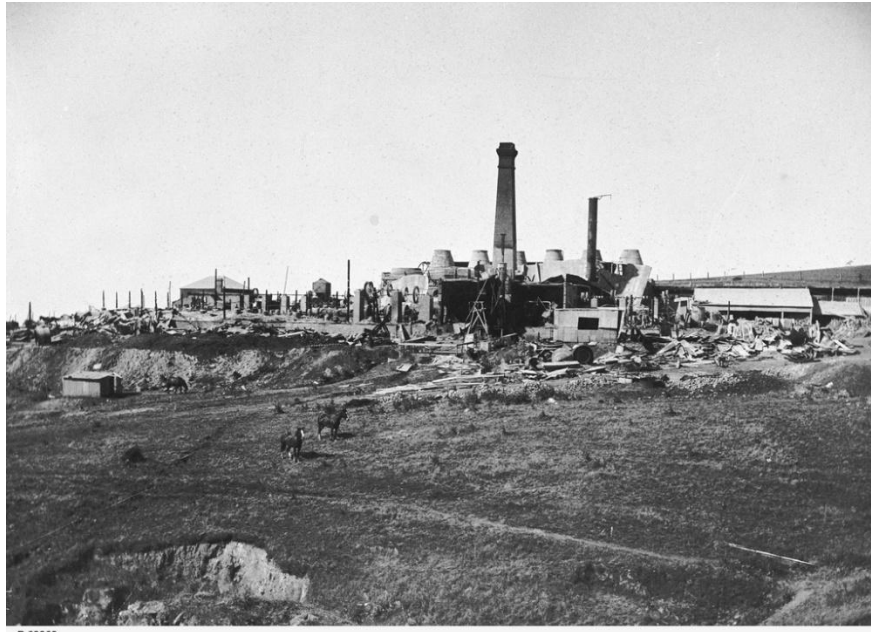
State Library of South Australia - Brighton Cement Company [B 60060], BRIGHTON: The ruins of Brighton Cement Company after destruction by fire; the main driving-shaft with its pulley-wheels can still be seen. 1909, Part of Brighton Collection.
